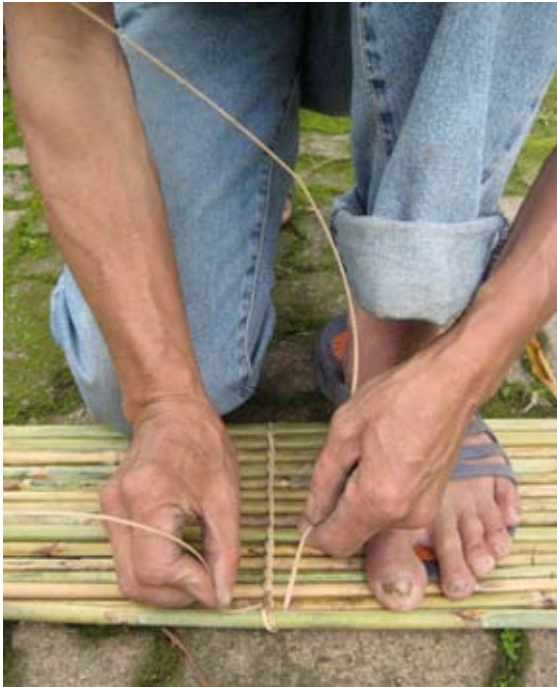
Binding runo reeds with rattan for use as ceiling panels. Winaca Village, June 11, 2007.
